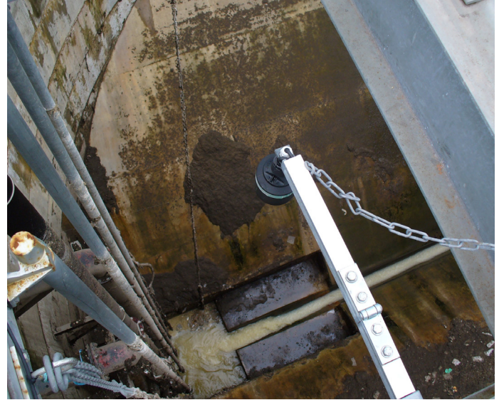
Another noisy wet well successfully measured by DATEM Echo Processing Software
