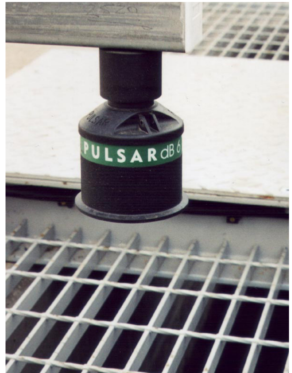
A dB6 transducer looking through a metal grid with the power of DATEM
