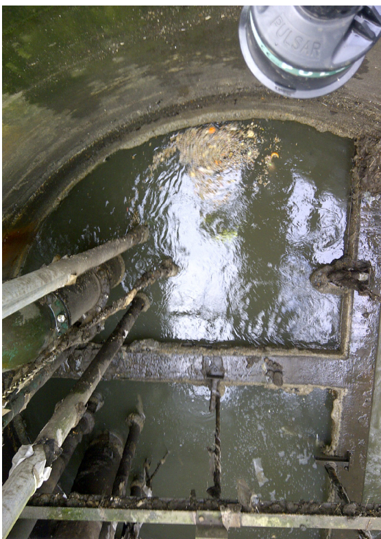
Example of a cluttered wet well
